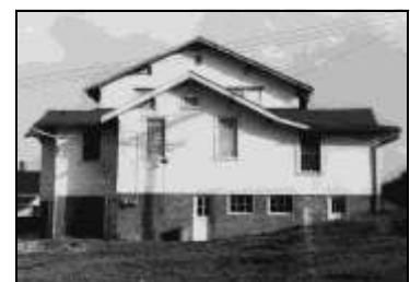
Back view of the Lucas Street church. New Sunday School rooms were added in 1950.
