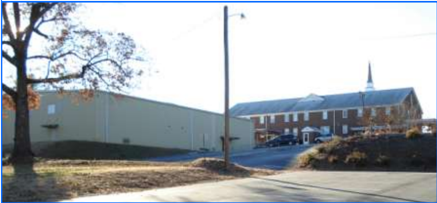
Our Family Life Center (activity building) as seen from the back of the church. It contains a full gymnasium, kitchen, dining area, classrooms, and large youth game/classroom/meeting room.
